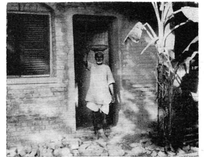
A south door is made into the large boarding room opening onto a recently completed long cement verandah. A day laborer carries cement for repair work.
