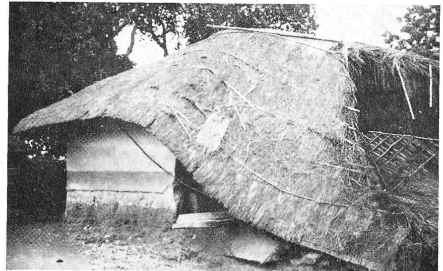
Floods washed away many houses, left others like this.
