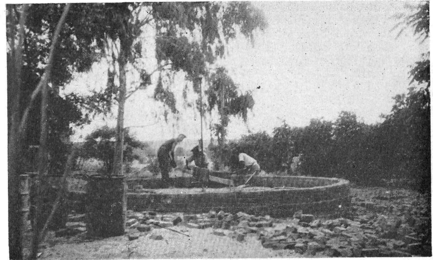
The Sikalongo water reservoir (tank) in construction
